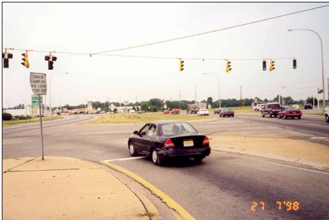
FIGURE 1 Example wide median intersection where left-turn traffic is separated from adjacent through traffic.
