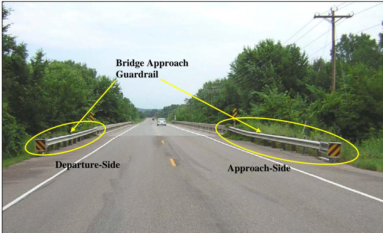
**FIGURE 1 County highway bridge with approach guardrail (Minnesota).**
