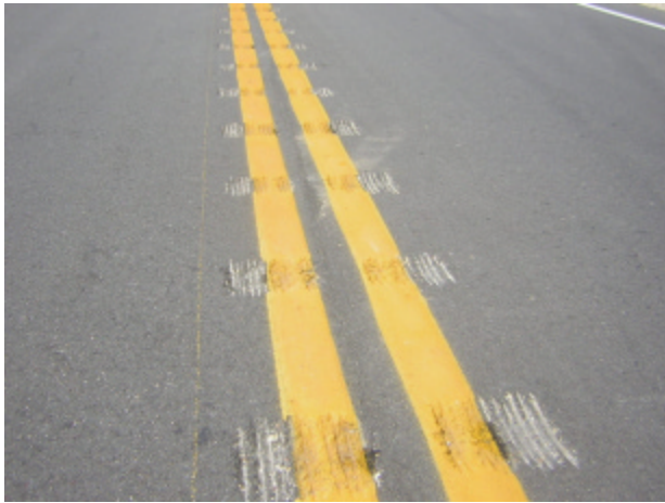
a. Alternative Pattern (2800 ft installed)
