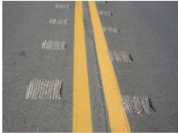
b. Standard Pattern (38,400 ft installed)
