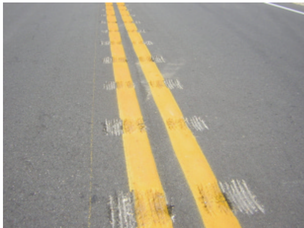
a. Alternative Pattern (2800 ft installed)
