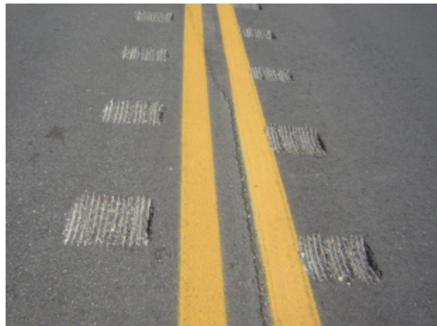
b. Standard Pattern (38,400 ft installed)
