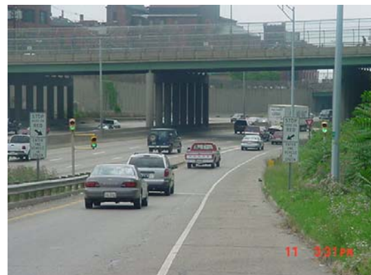
Figure 1-2. Typical Freeway Ramp Meter Deployment 2
