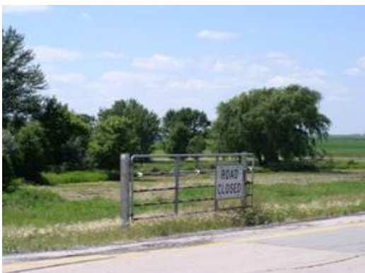
Figure 1-17. I-90 Ramp Gate 6
