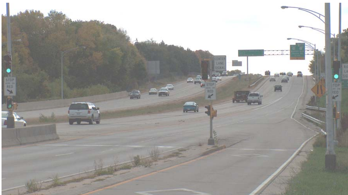
Figure 2-2. Eastbound Beltline Ramp Meter at Whitney Way
