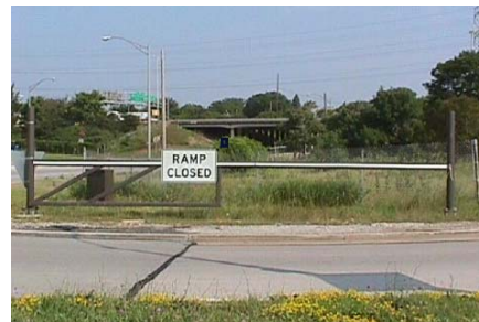
Figure 1-7. Horizontal Swing Arm Traffic Gate 3
