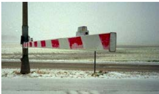
Figure 1-18. Iowa Ramp Closure Gate
